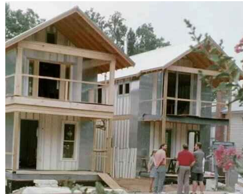
KATRINA HOMES-BUILT AFTER HURRICANES THERMASTEEL PANELS
