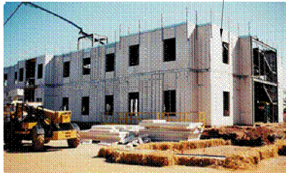
HOTEL COMPLEX DURING CONSTRUCTIONS THERMASTEEL PANELS
