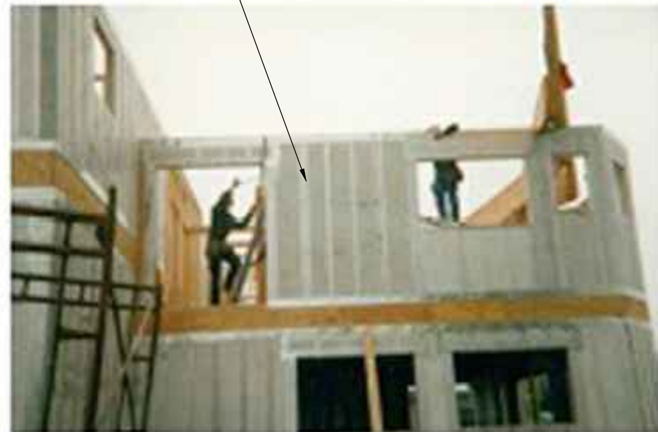
TYPICAL HOUSE CONSTRUCTION ON THERMASTEEL PANELS
