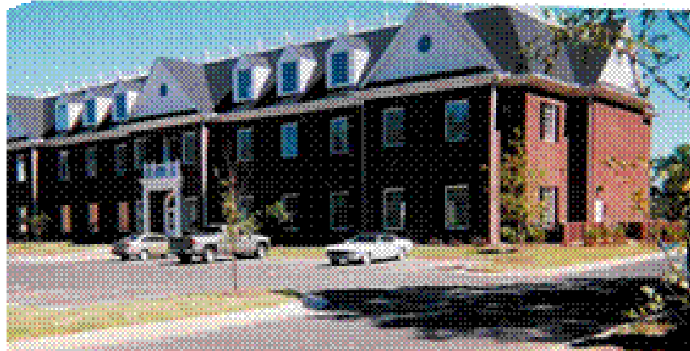
COMPLETED HOTEL COMPLEX THERMASTEEL PANELS
