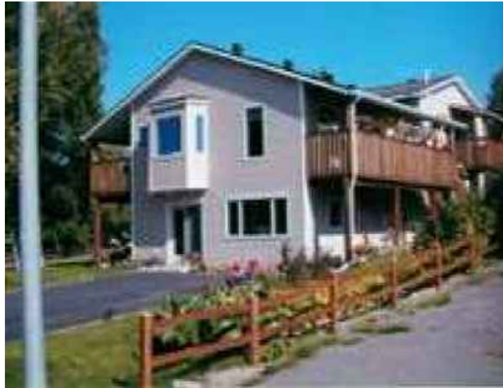
COMPLETED ANCHORAGE HOUSE THERMASTEEL PANELS
