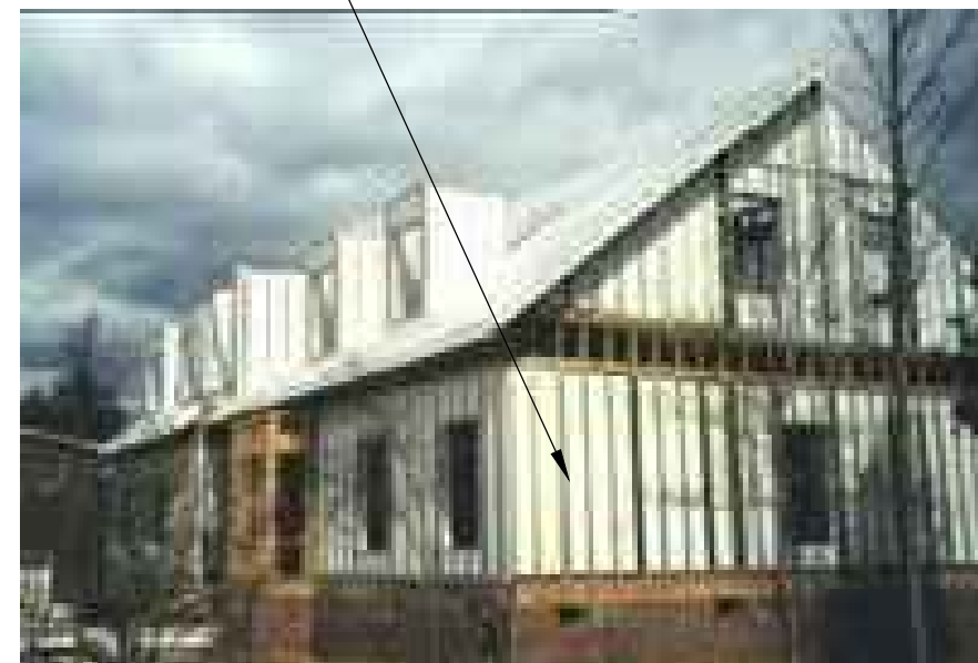
HOUSE DURING CONSTRUCTION THERMASTEEL PANELS
