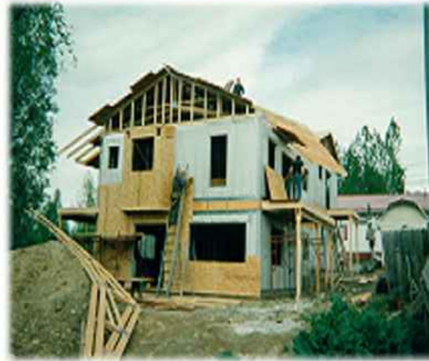
ANCHORAGE HOUSE DURING CONSTRUCTION ON THERMASTEEL WALL AND ROOFING PANELS
